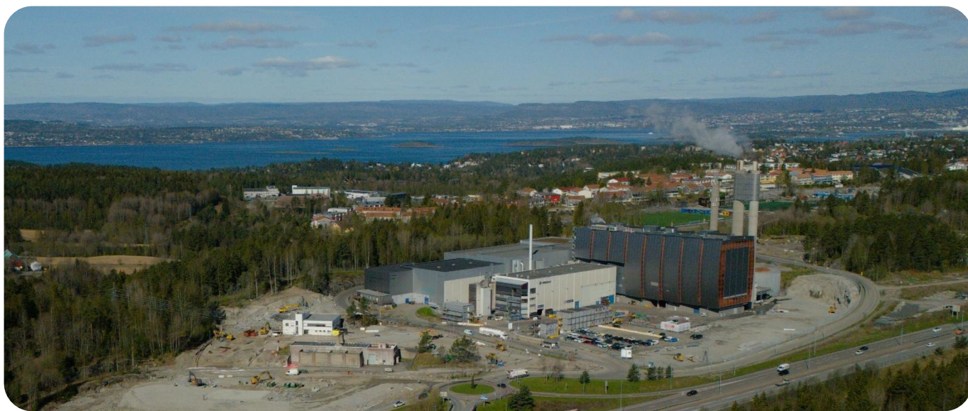
A photograph of Hafslund Celsio’s Klemetsrud facility. Photograph by Hafslund Celsio team.
